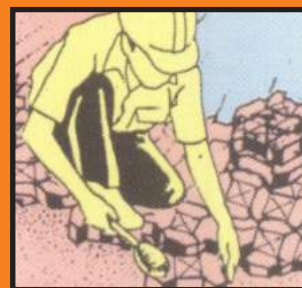
LAY AND INTERLOCK PAVER BLOCKS
